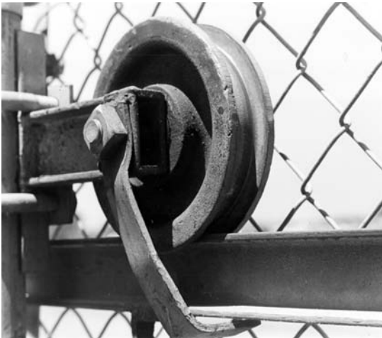
Figure 20 Too much play between rollers and rails
