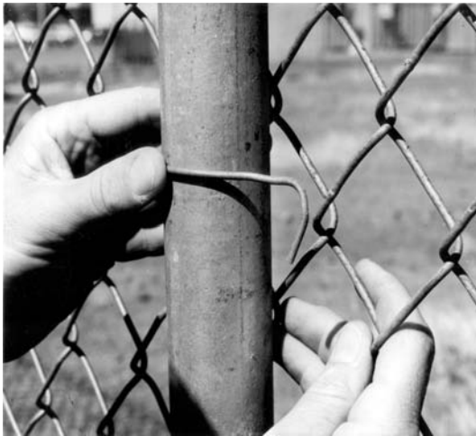
Figure 12 Loose fabric at fence posts or horizontal rails
