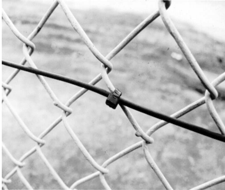
Figure 26. Cable Tie Installation
