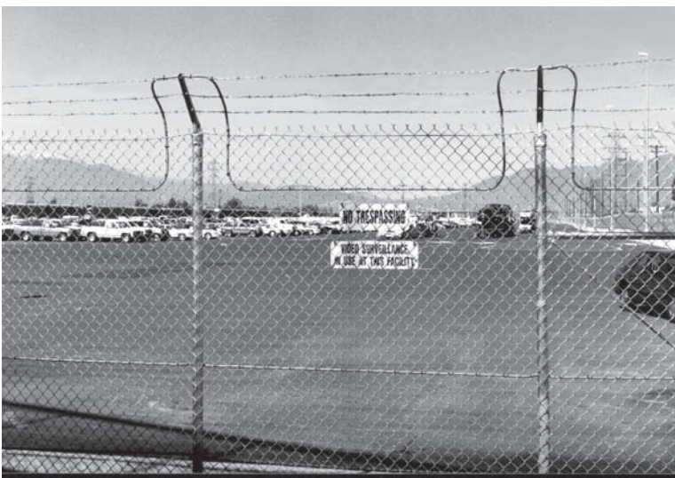
Figure 27. Barbed wire Outrigger
