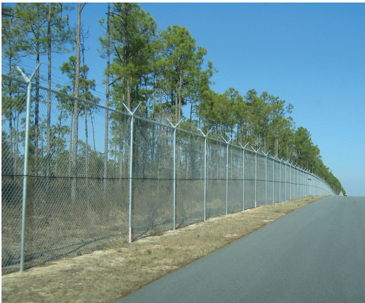
Example of FiberPatrol along a perimeter fence
