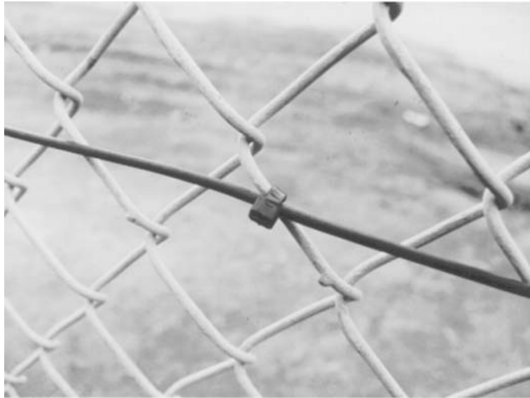
Figure 16. Cable Tie Installation
