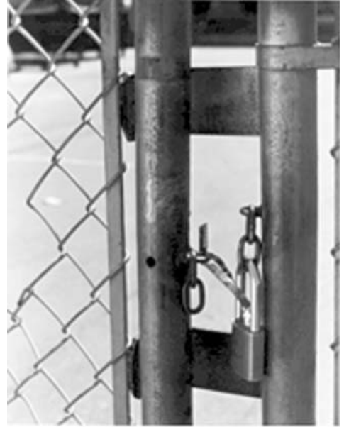
Figure 9 Chain and lock free to vibrate against gate
